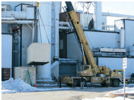
A crane was used to place two shipping containers near the steam plant. These containers house the equipment used to conduct further experiments under the CO 2 (CACHYS) project.
