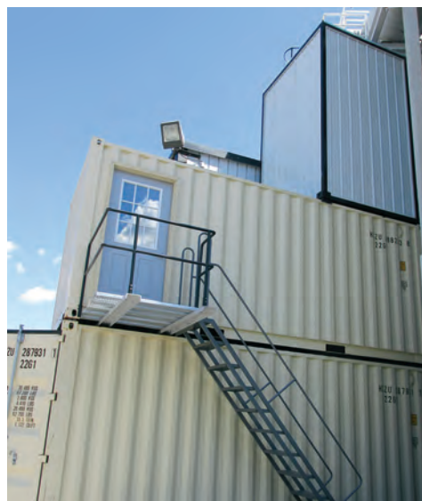
Once assembled, the portable lab has three levels. The stair case leads to the office which is insulated and separate from the lab area for the instrumentation and controls for the portable lab. The bottom container houses the tools and necessary parts to operate the portable lab.
